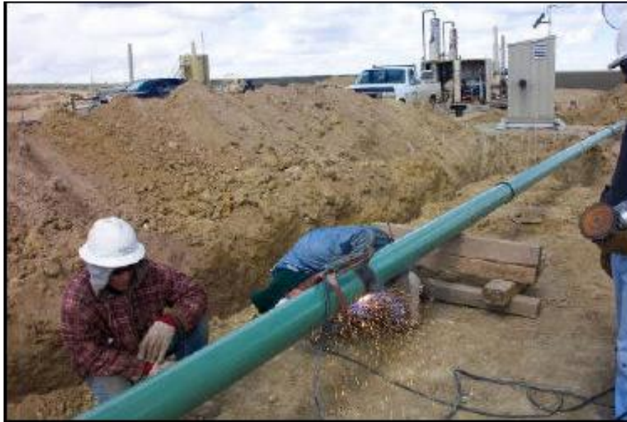
Gas-line construction (pinedaleonline.com)
